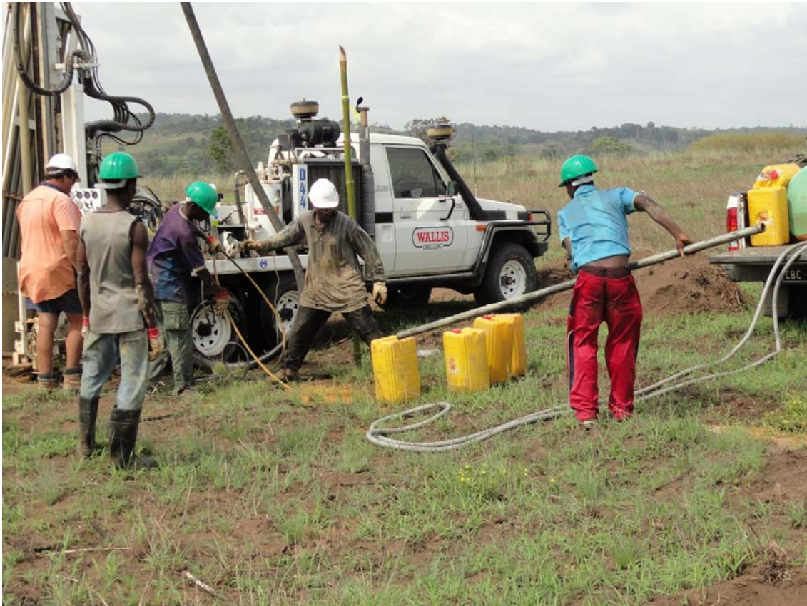
Figure 2-2 Aircore Drilling Cabinda Phosphate Project
