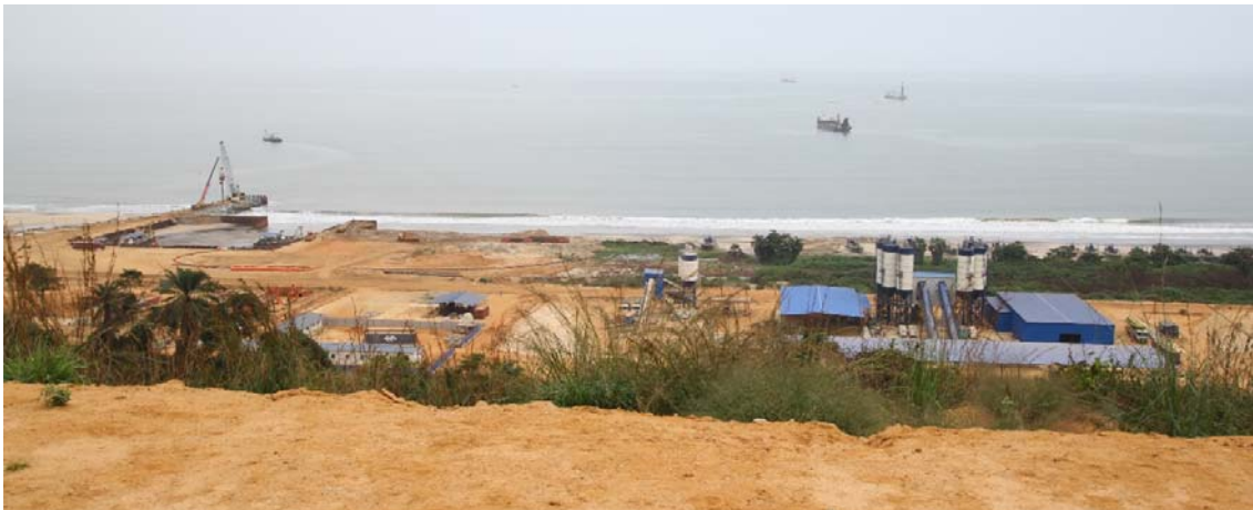
Figure 7-1 Material Offload Facility (MOF) under construction Porto de Caio 2017
