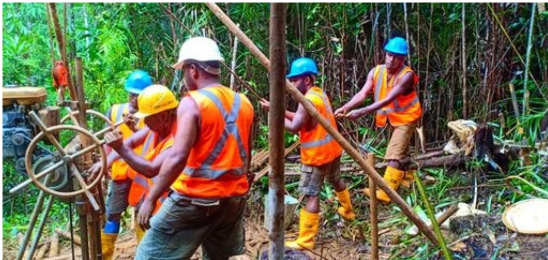
Picture 1. Drilling in progress at Jejovo
