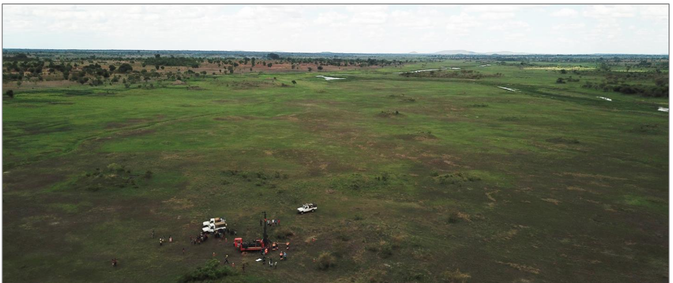
Figure 10. 2019 air-core drilling at Bua Channel.
