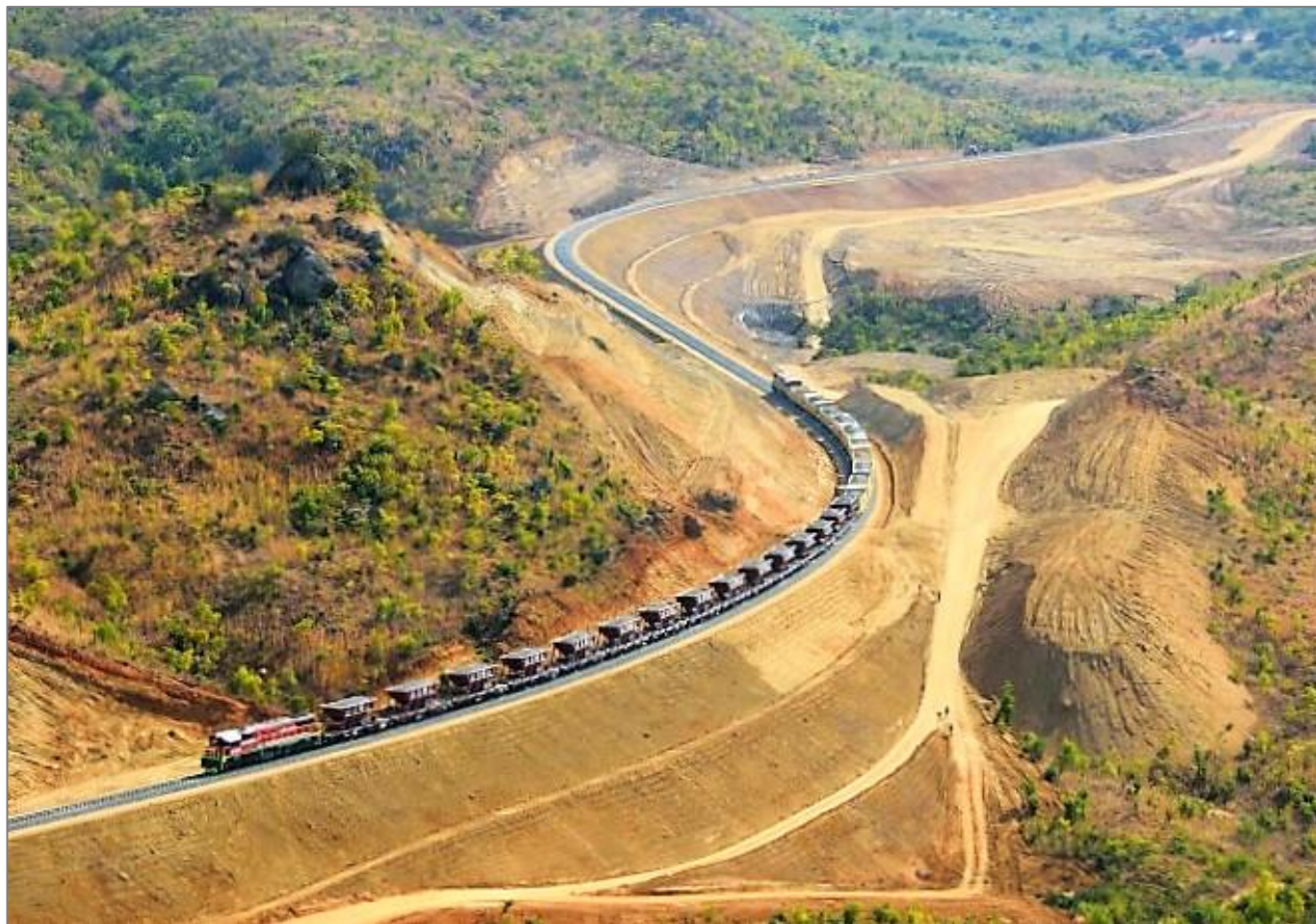
Figure 2: Nacala Logistics Corridor in Operation
