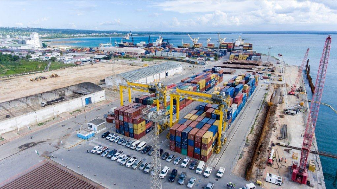
Figure 4: Container storage and loading facilities at the port of Nacala
