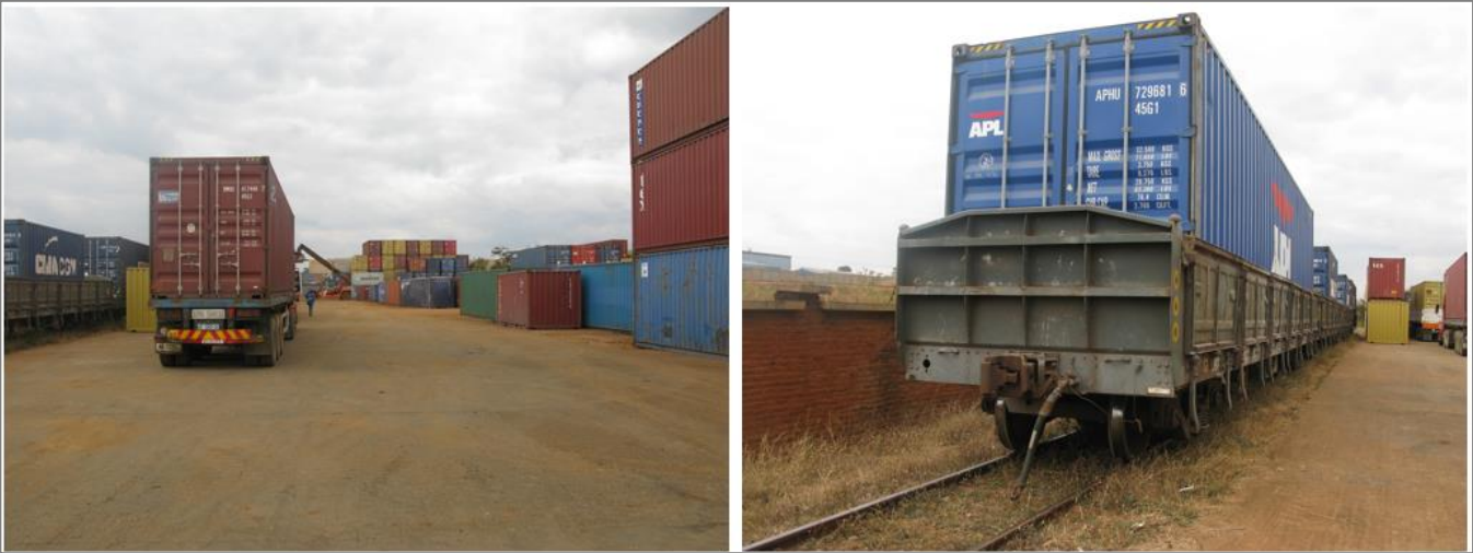
Figure 5 and 6: Container storage, loading and operating rail facilities at Kanengo (Lilongwe)
