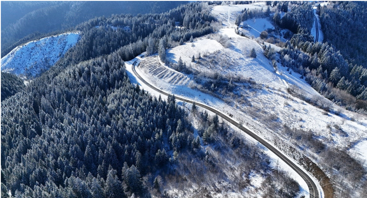
Figure 14: Aerial view of the completed road, December 2023
