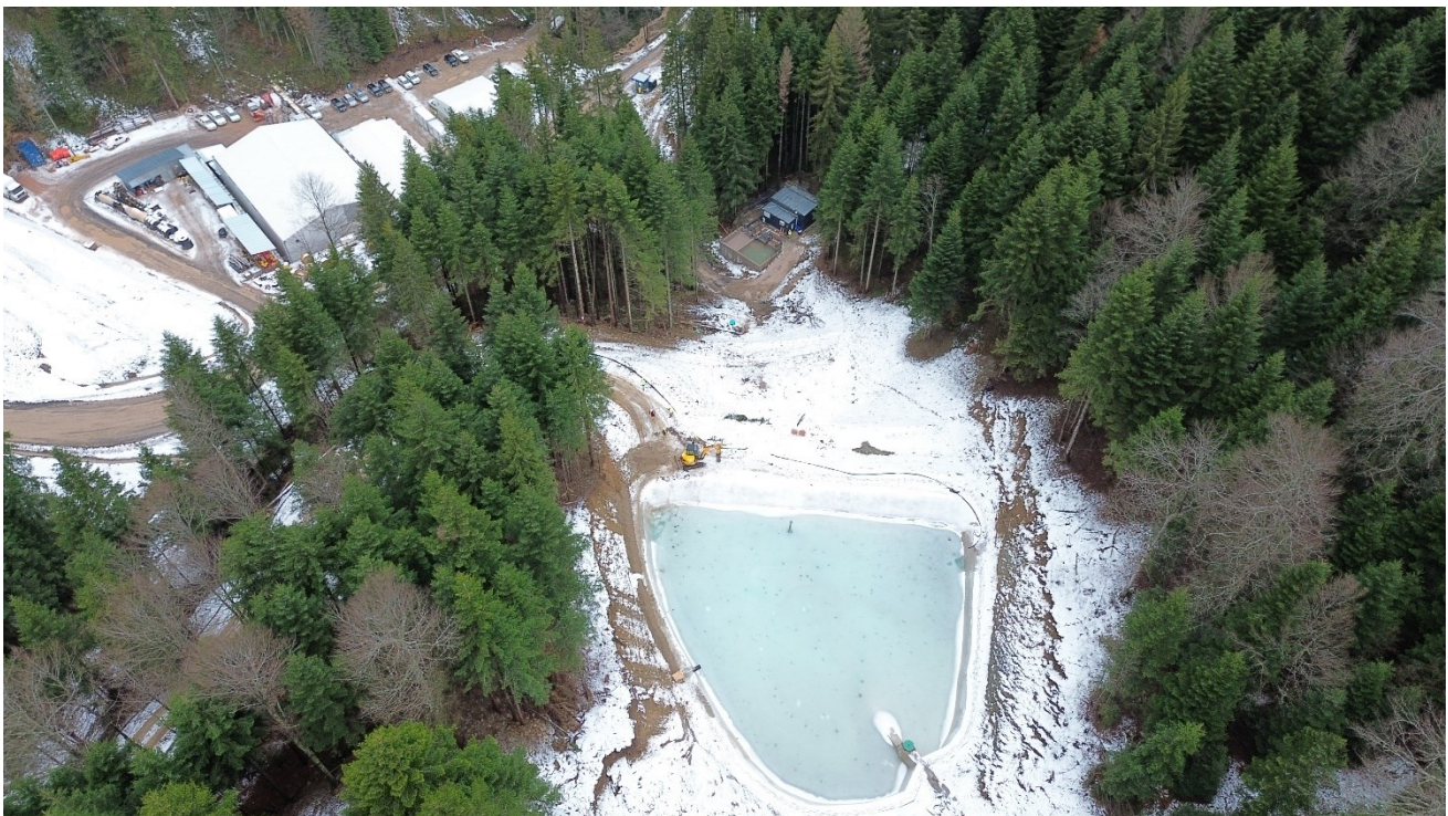
Figure 7: Water Treatment Plant, December 2023
