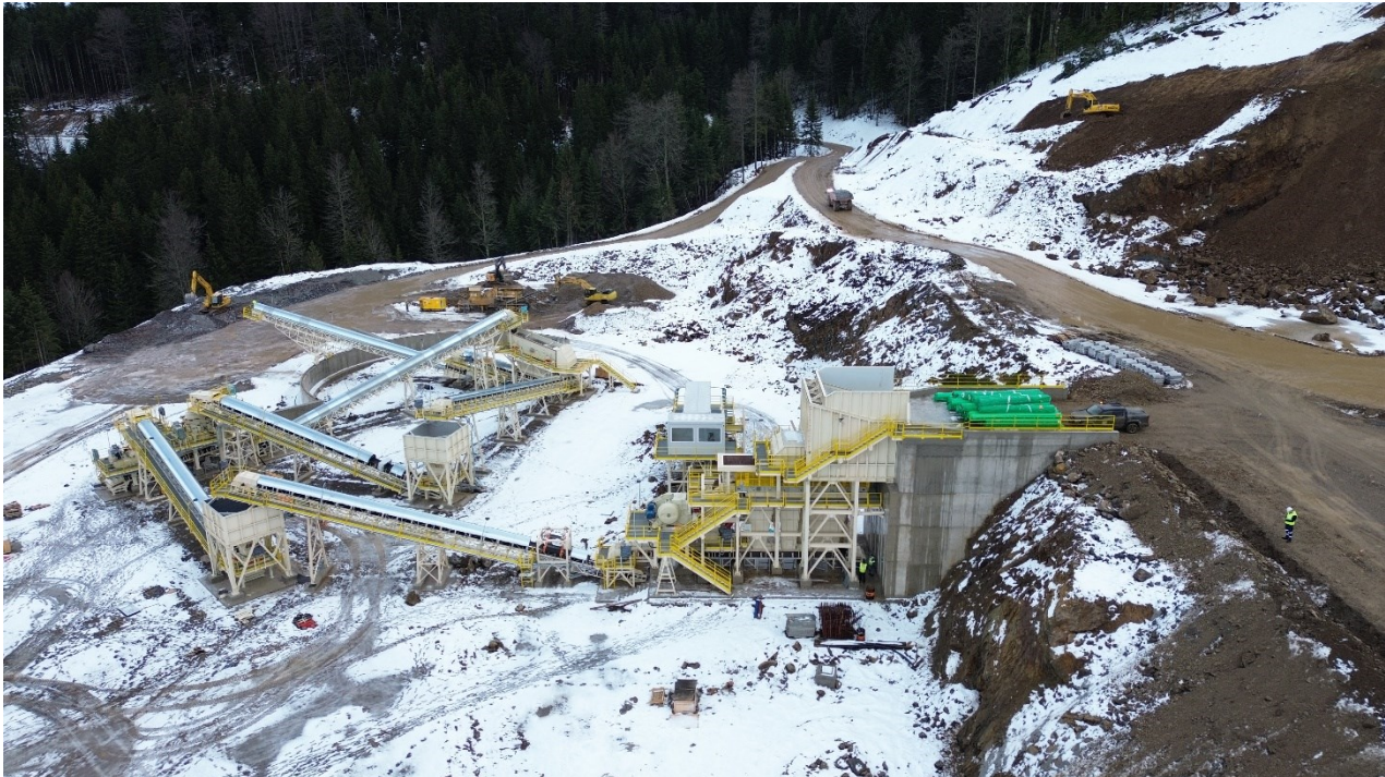
Figure 8: Crusher Plant, December 2023
