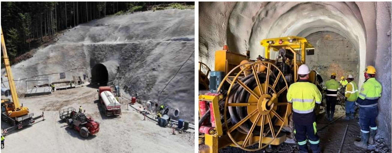
Lower Decline Portal and Underground Development (July 2022)
