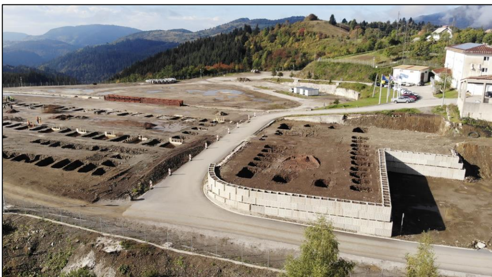
Figure 4: Vares Processing Plant (September 2022)
