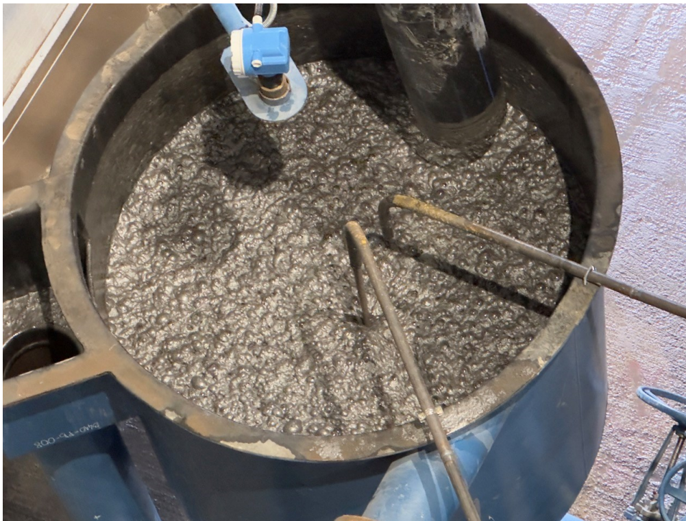
Figure 1: Pump box, 27 February 2024
