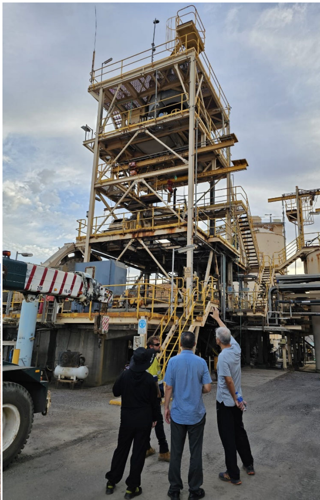
Figure 3: Sundry representatives inspecting refurbishment at Paulsens
