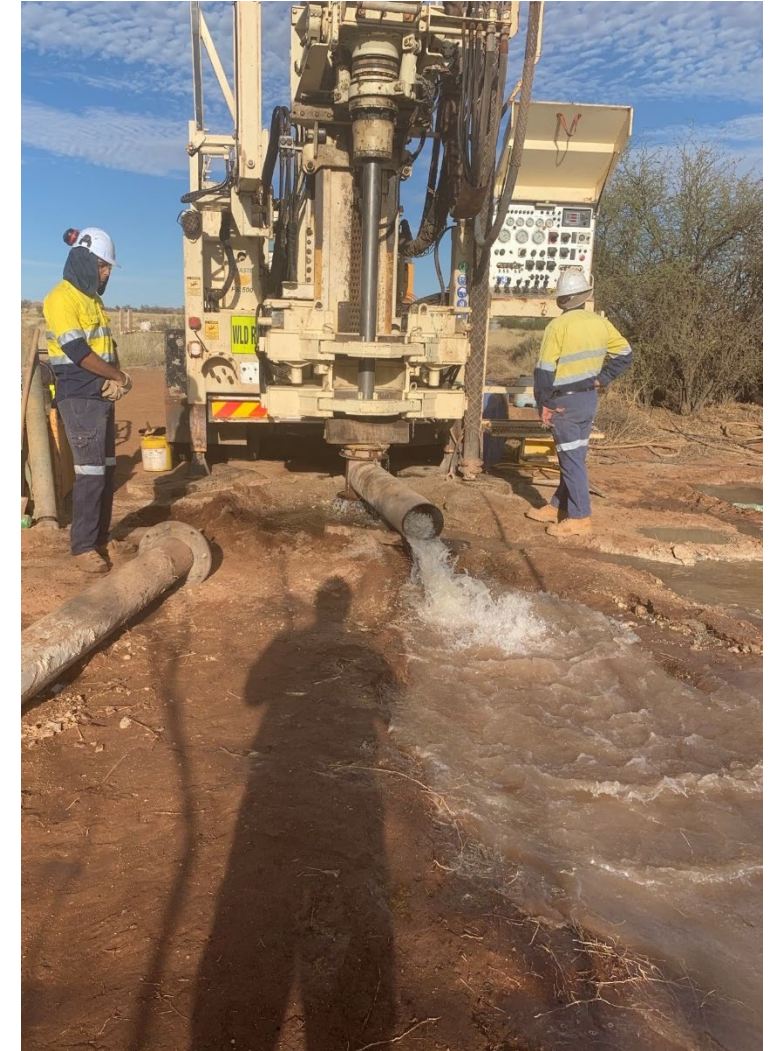
Water bore construction and testing
