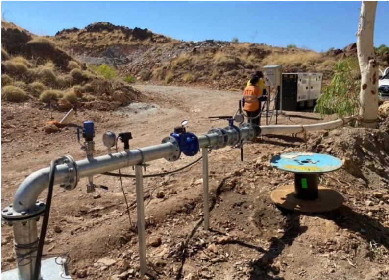
Bore field installation
