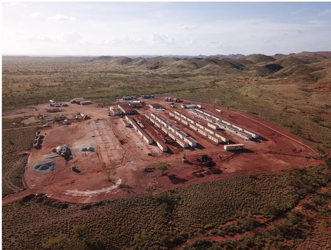
Figure 3: Warrawoona site layout looking North East
