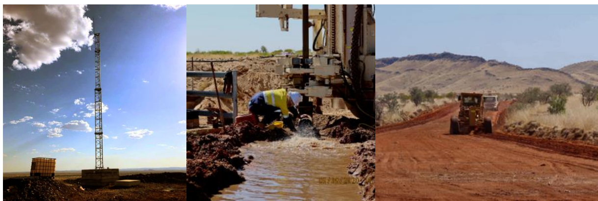
Figure 4: Telecommunications Towers, Bores and Access Road Completed
