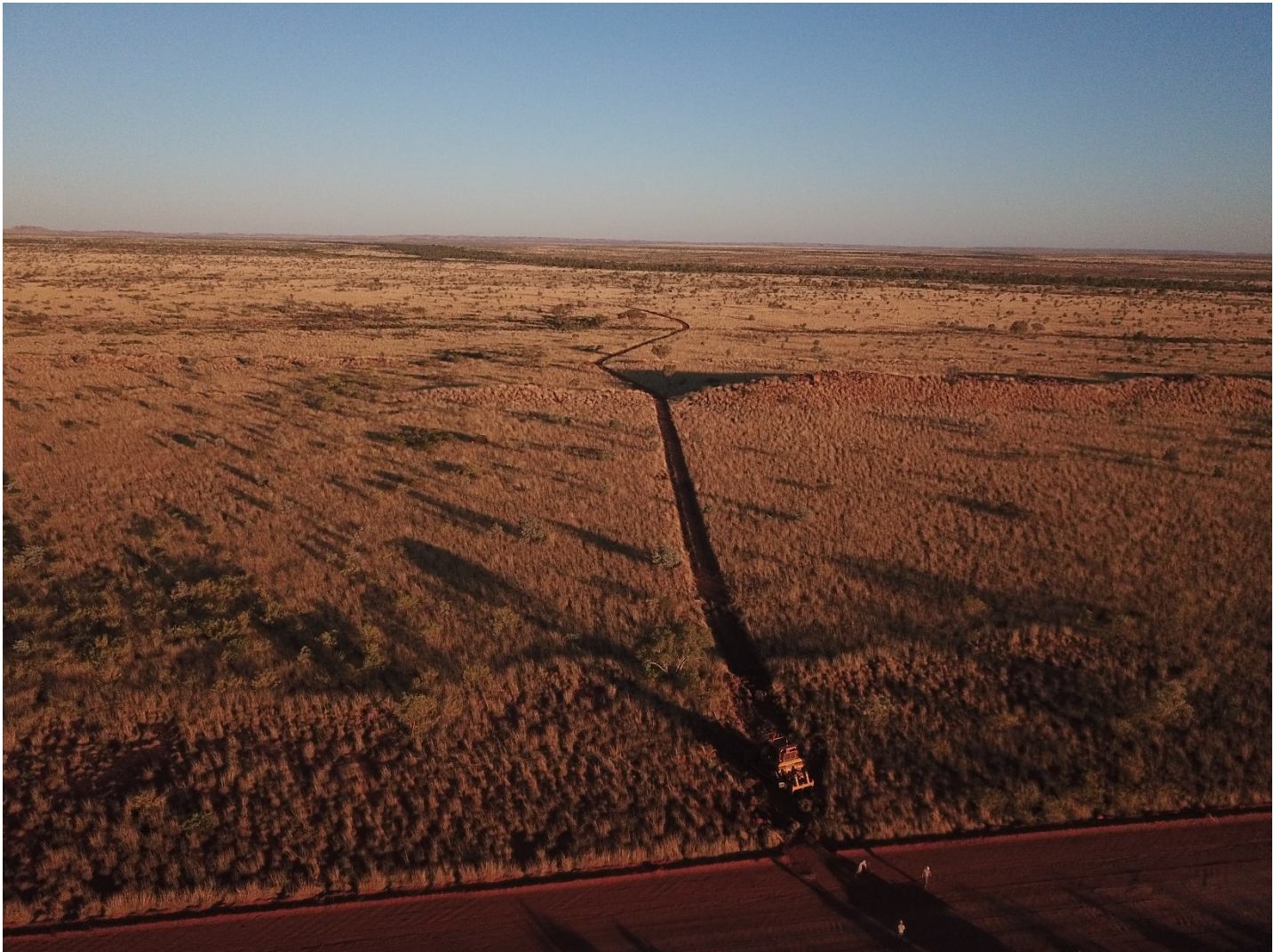
New access road construction commenced
