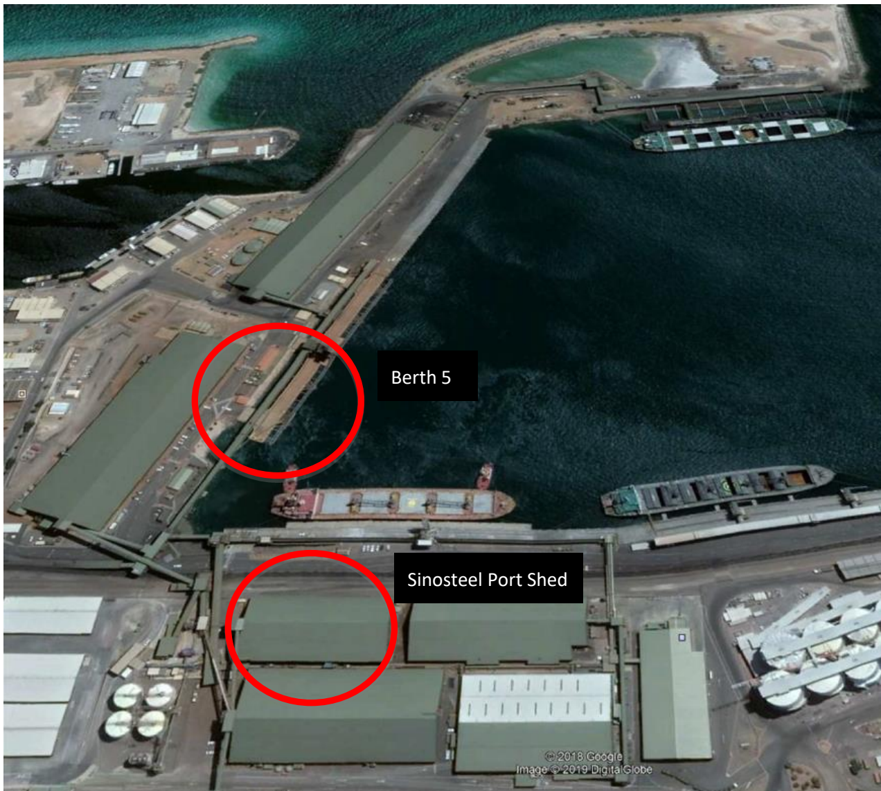
Existing Geraldton Port Infrastructure showing location of Sinosteel Port Shed and the Multi-user bulk shipping loading facility (Berth 5)
