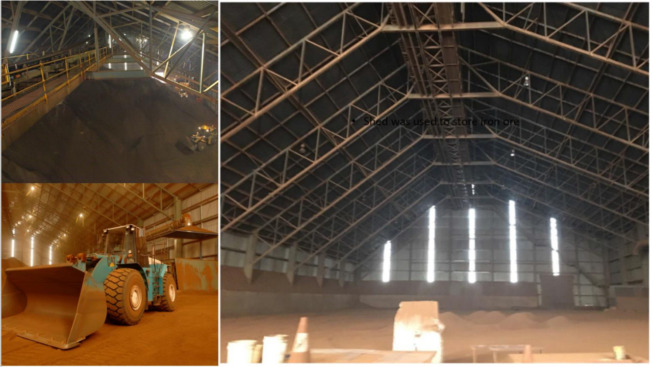
Existing Sinosteel Port Shed – internal view
