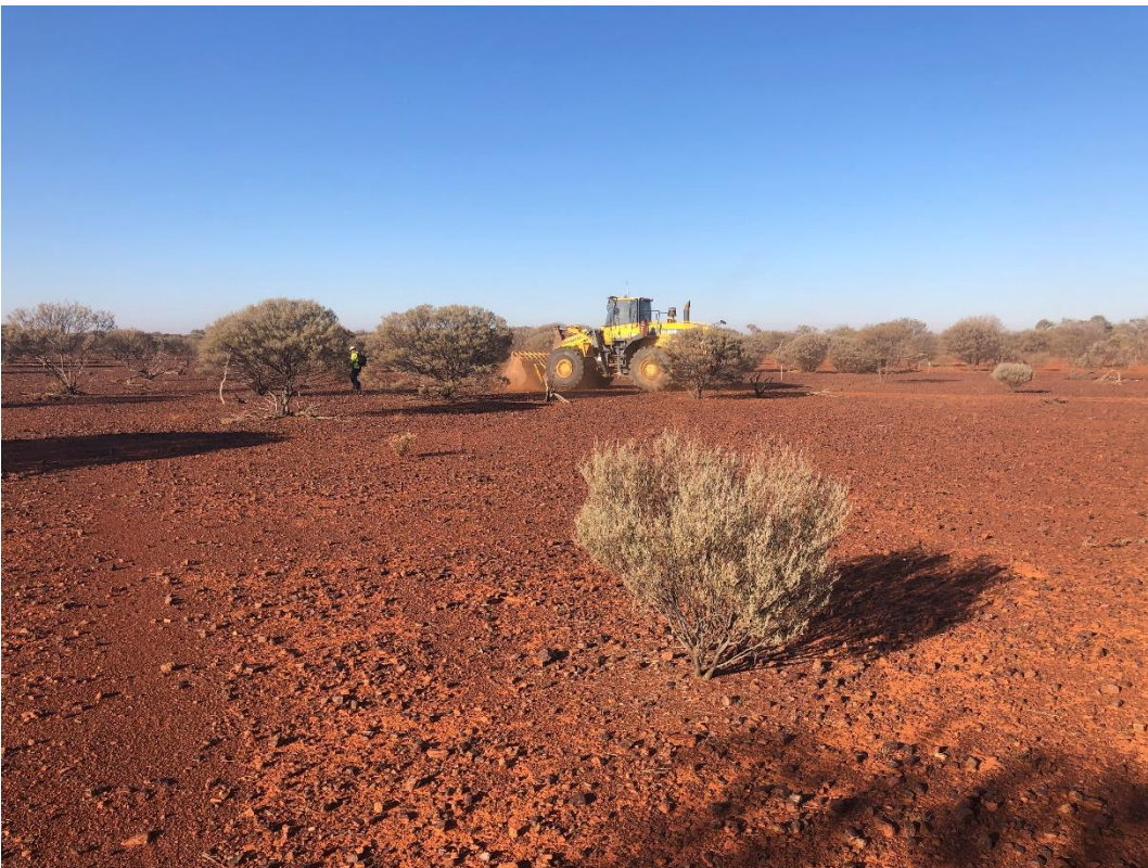
Clearing activities – Iron Ridge Project
