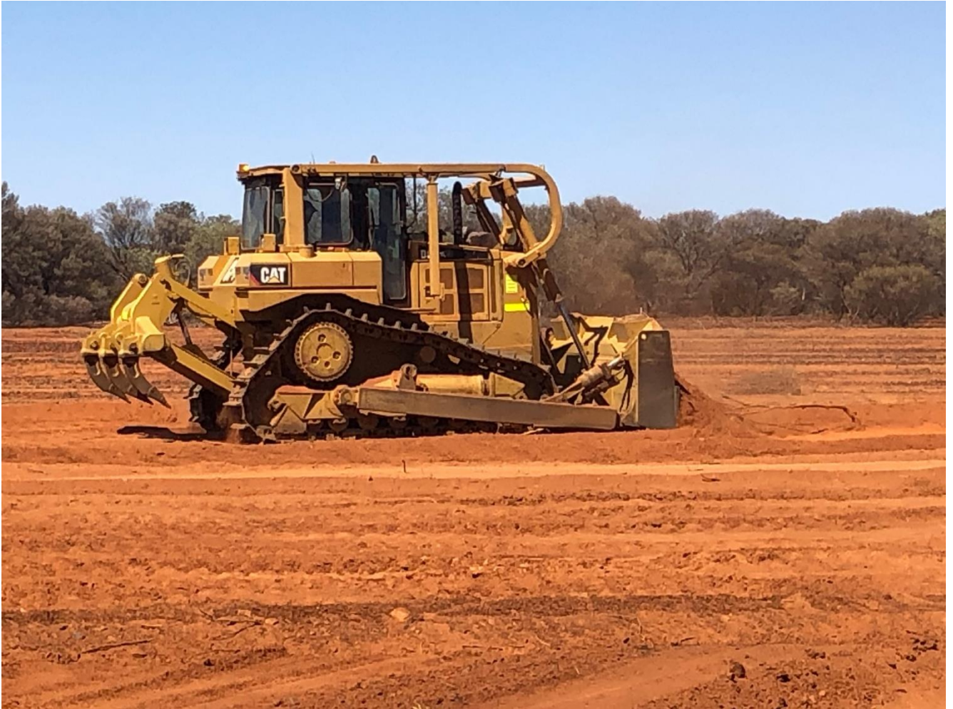
Topsoil stripping – Iron Ridge Project
