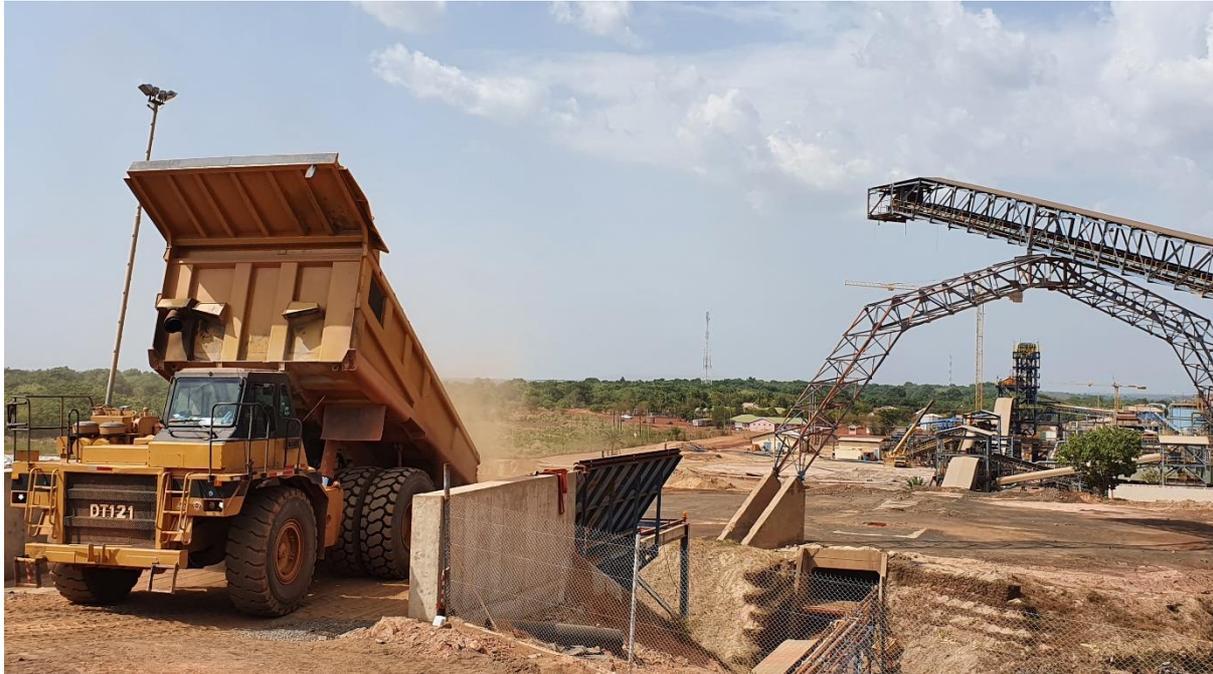
**Figure 3: Truck direct loading to the oxide circuit dump pocket during commissioning.**
