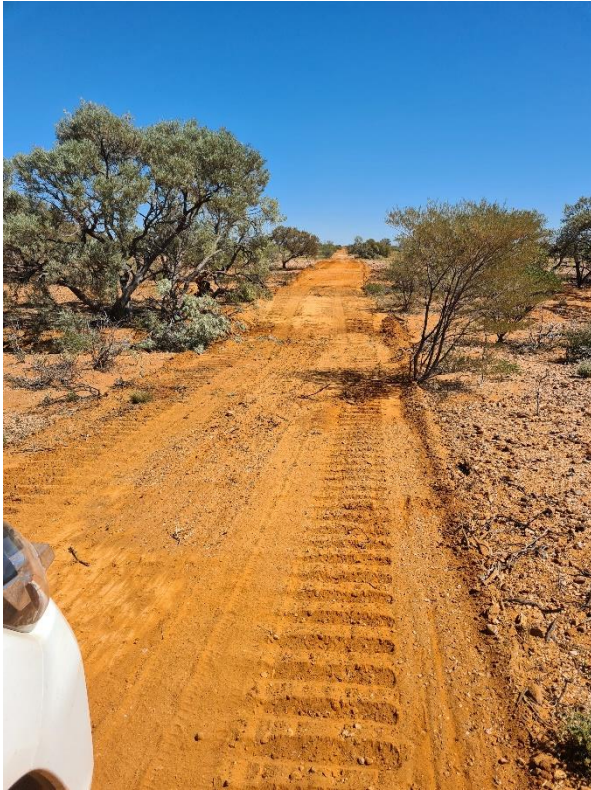
Figure 3: Access track construction
