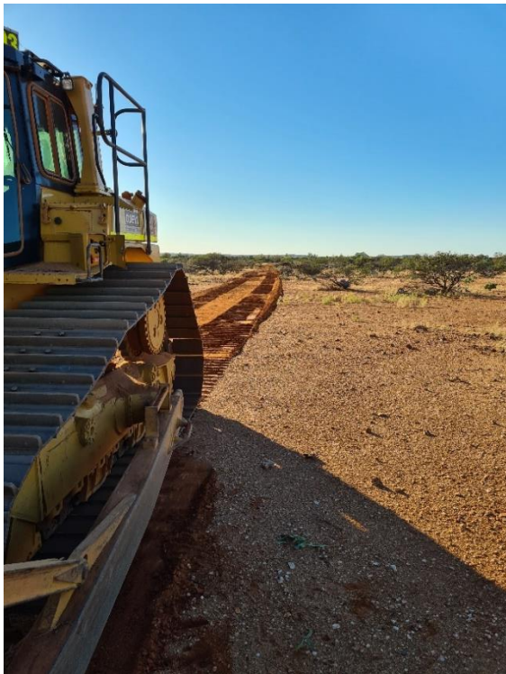
Figure 5: Site access track clearing
