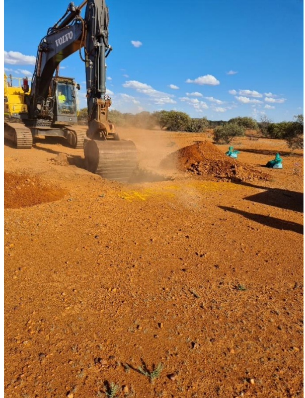
Figure 4: Geotechnical test pitting
