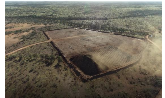
Figure 6. First blast successfully completed and ready for excavation.
