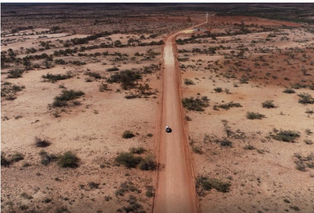
Figure 1: Site Access Road
