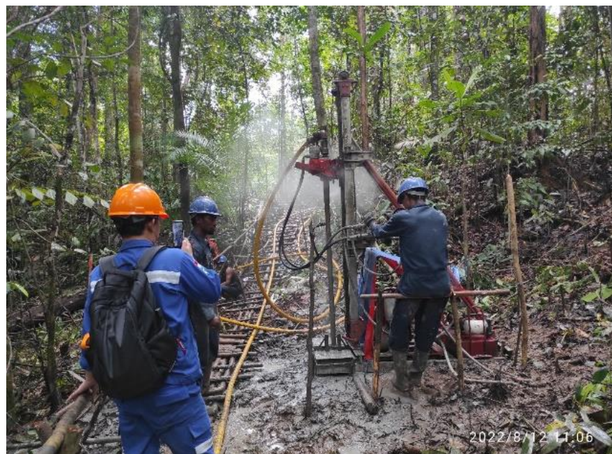
Photo 1: Compressor shot hole drilling operations
