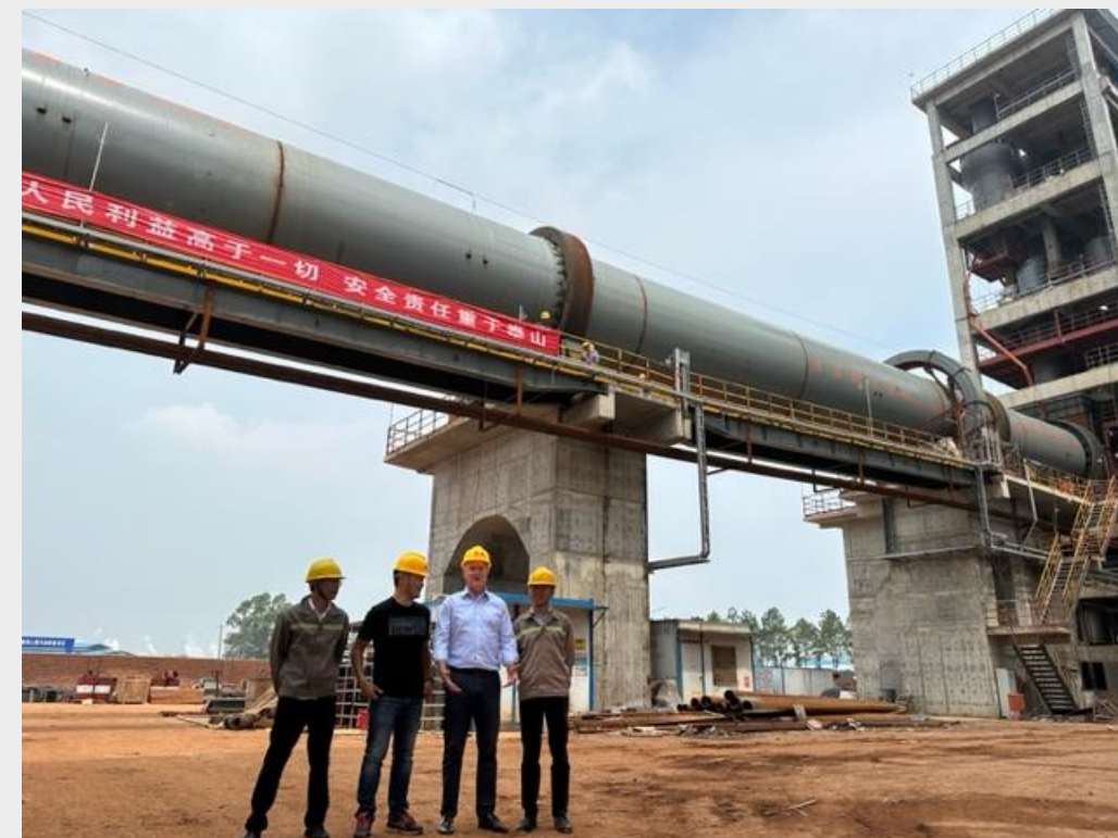
Leo and Ganfeng reps inspecting Ganfeng's new lithium hydroxide converter at Fengcheng, Jiangxi in May 2023
