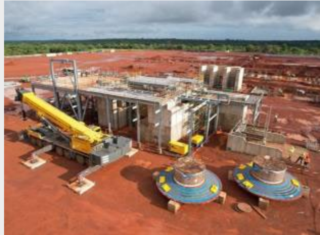
450 t crane in position for mill installation
