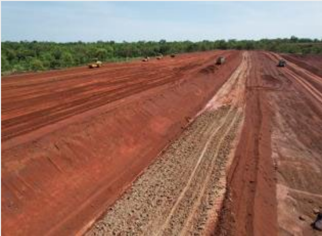
TSF embankment construction
