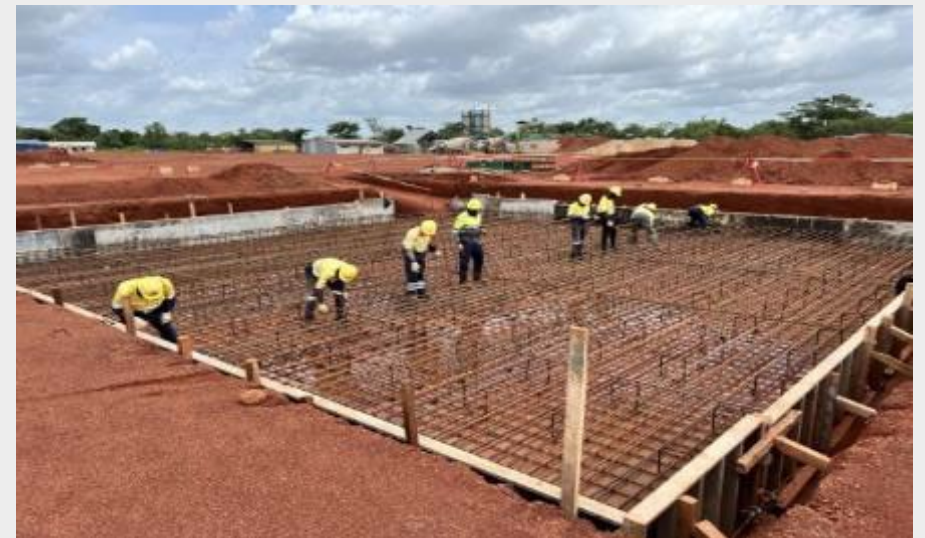
Ball mill site (top), steel fixing in Aug 2023 (below)
