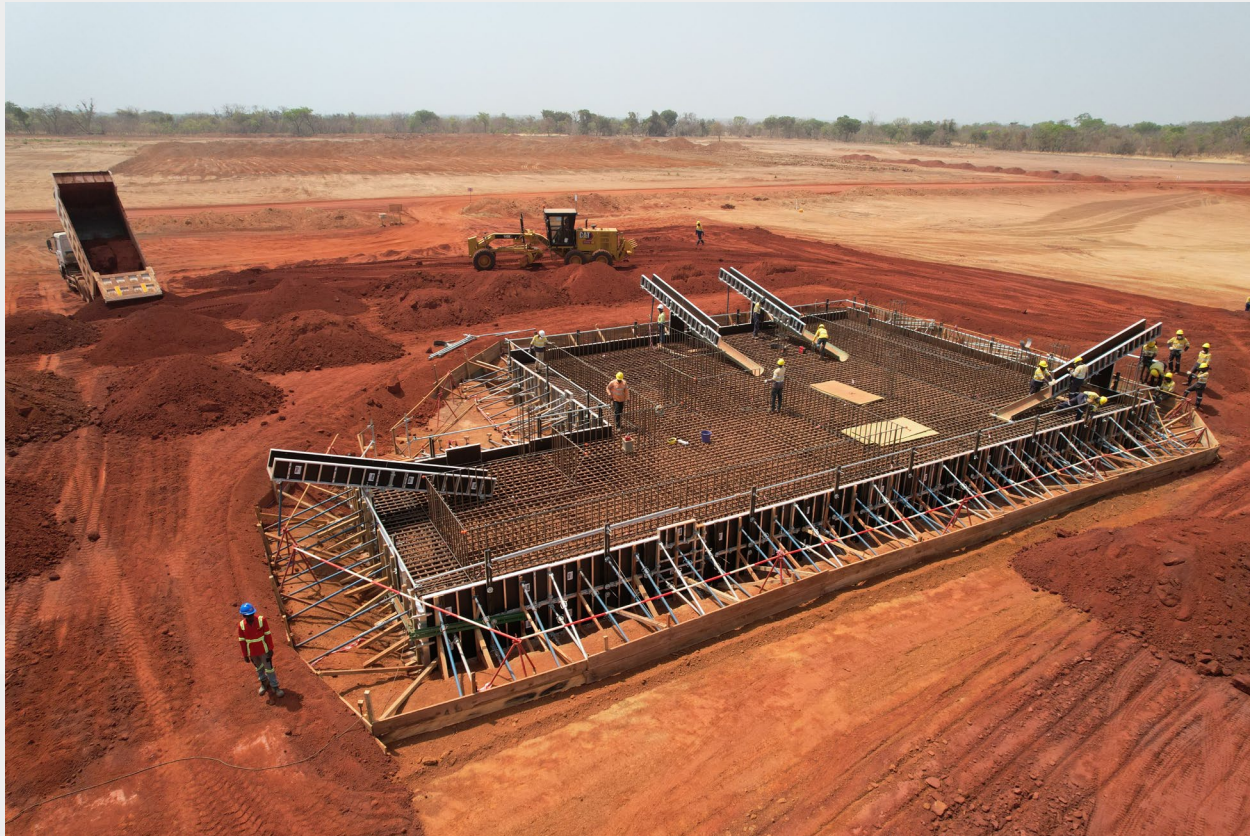
Ball mill raft slab preparations
