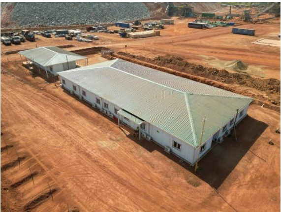
Figure 5: Plant administration office
