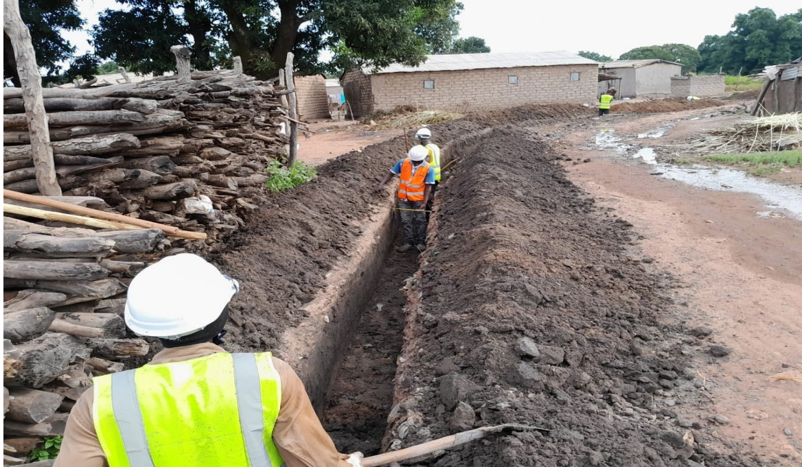
Image 12 - Commencement of the water supply project in Goulamina village
