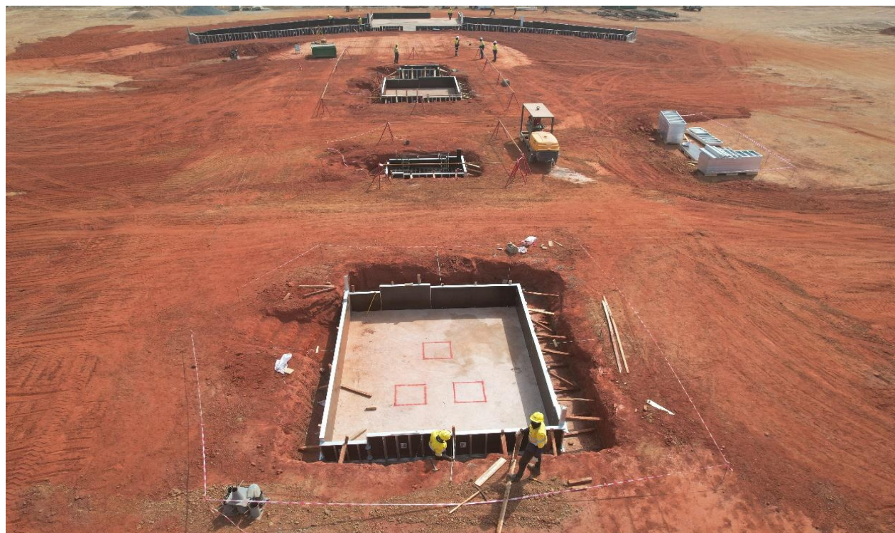
Image 3 - Primary crusher and conveyor concrete foundations poured during Q1 2023
