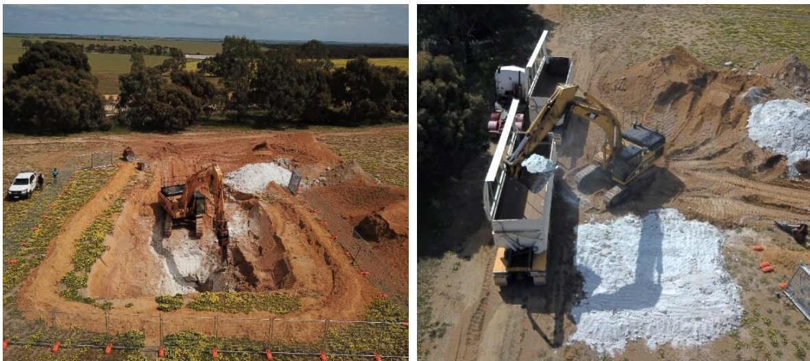
Figure 6: Test-pit in progress
