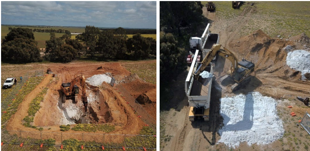
Figure 1: Test-pit in progress
