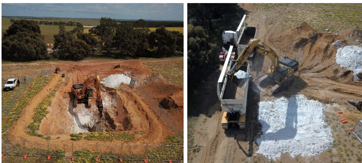
Figure 8: Test-pit in progress
