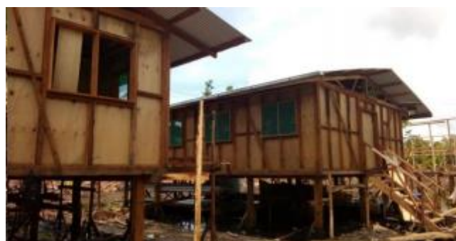
Camp construction underway utilising local carpenters and locally milled timber.
