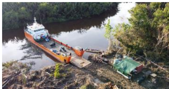
Barge unloading to commence earthworks.
