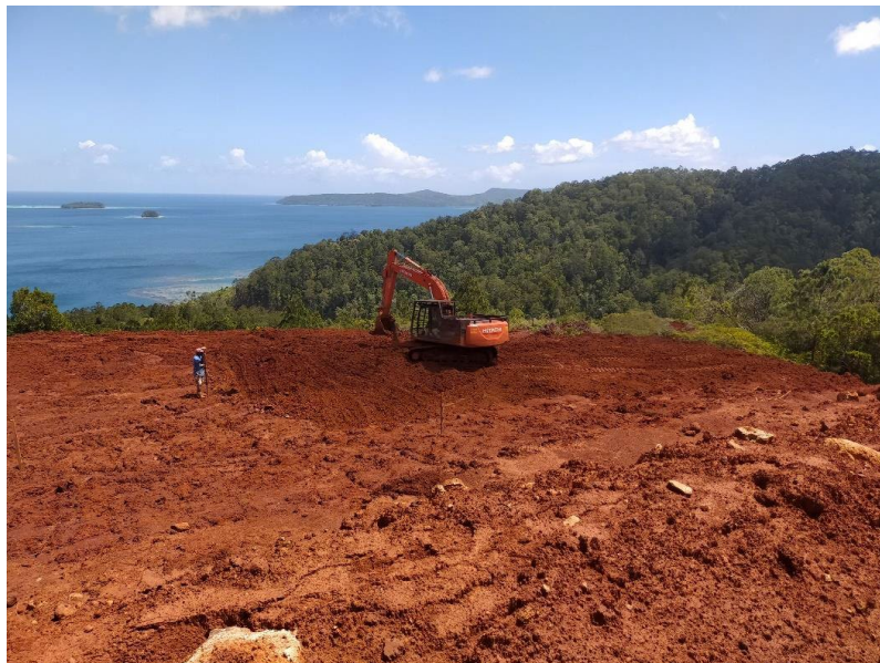
Photo: Stockpile Pad being prepared
