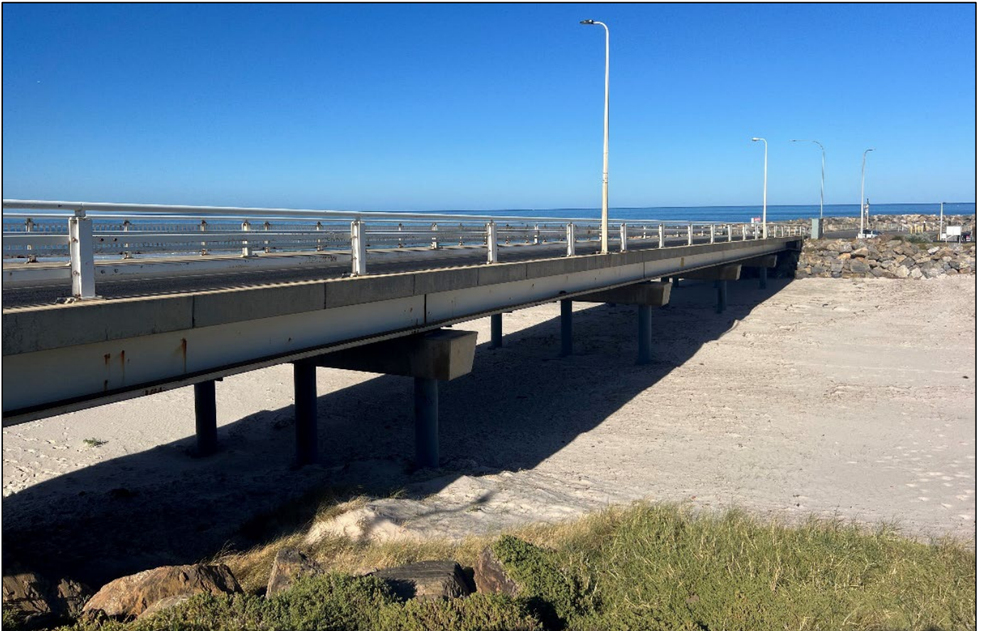
Figure 1: Trial infrastructure at West Beach Bridge, Adelaide, SA
