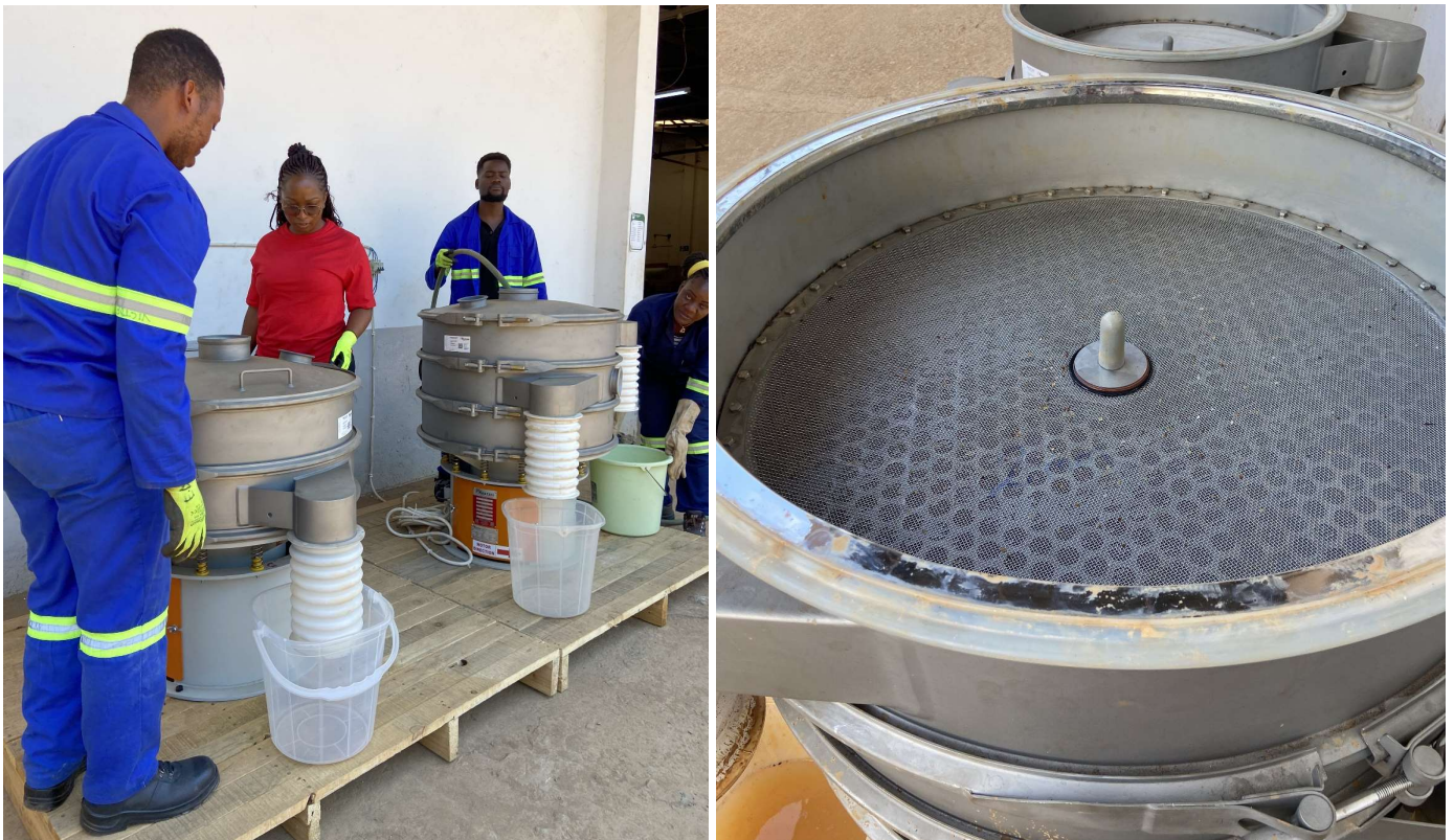
Figure 2. Installation of the new Kwatani 30-inch single-deck and double-deck vibrating separators for sizing and de-sliming bulk samples at the Company's Malawi laboratory and metallurgical facility
