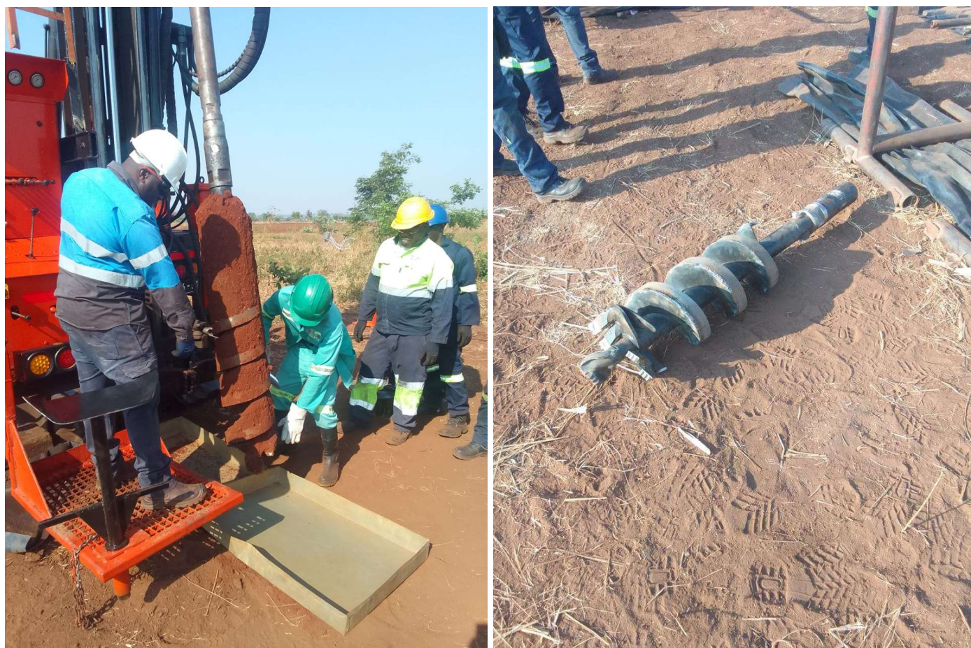
Figure 1. Mechanised drill with custom-made 300mm diameter spiral auger
