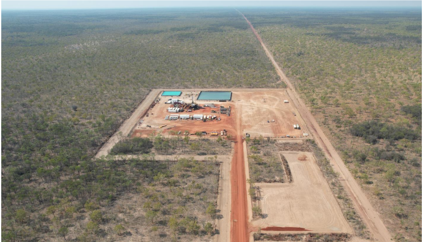
Figure 2: Well pad and preparation for the drilling of Amungee 2H in EP 98
