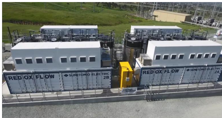
Sumitomo Electric's VRFB in San Diego, California
