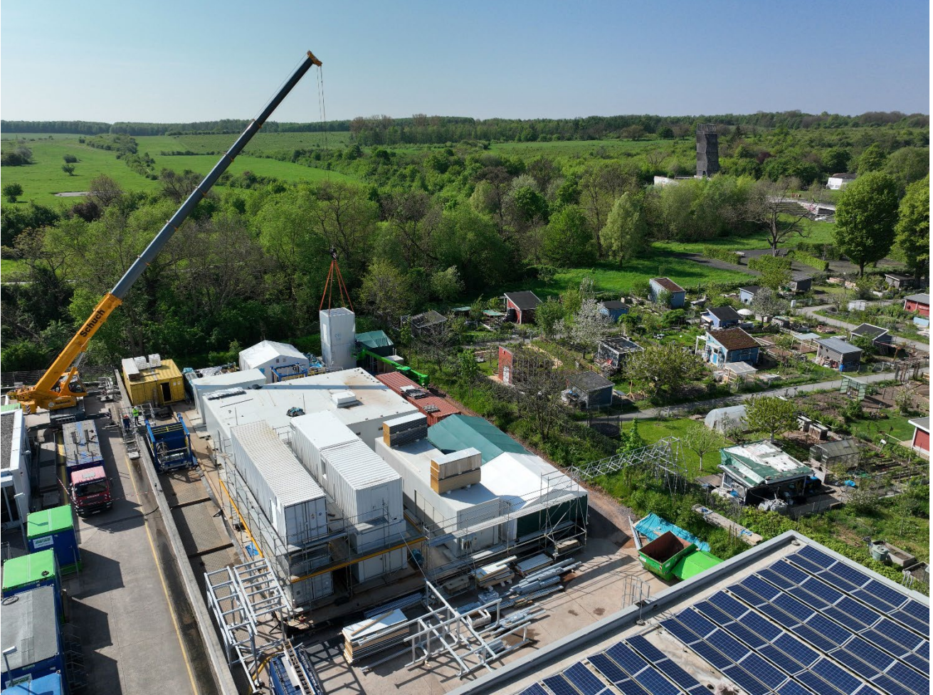
Figure 1: Vulcan's LEOP Plant, under construction
