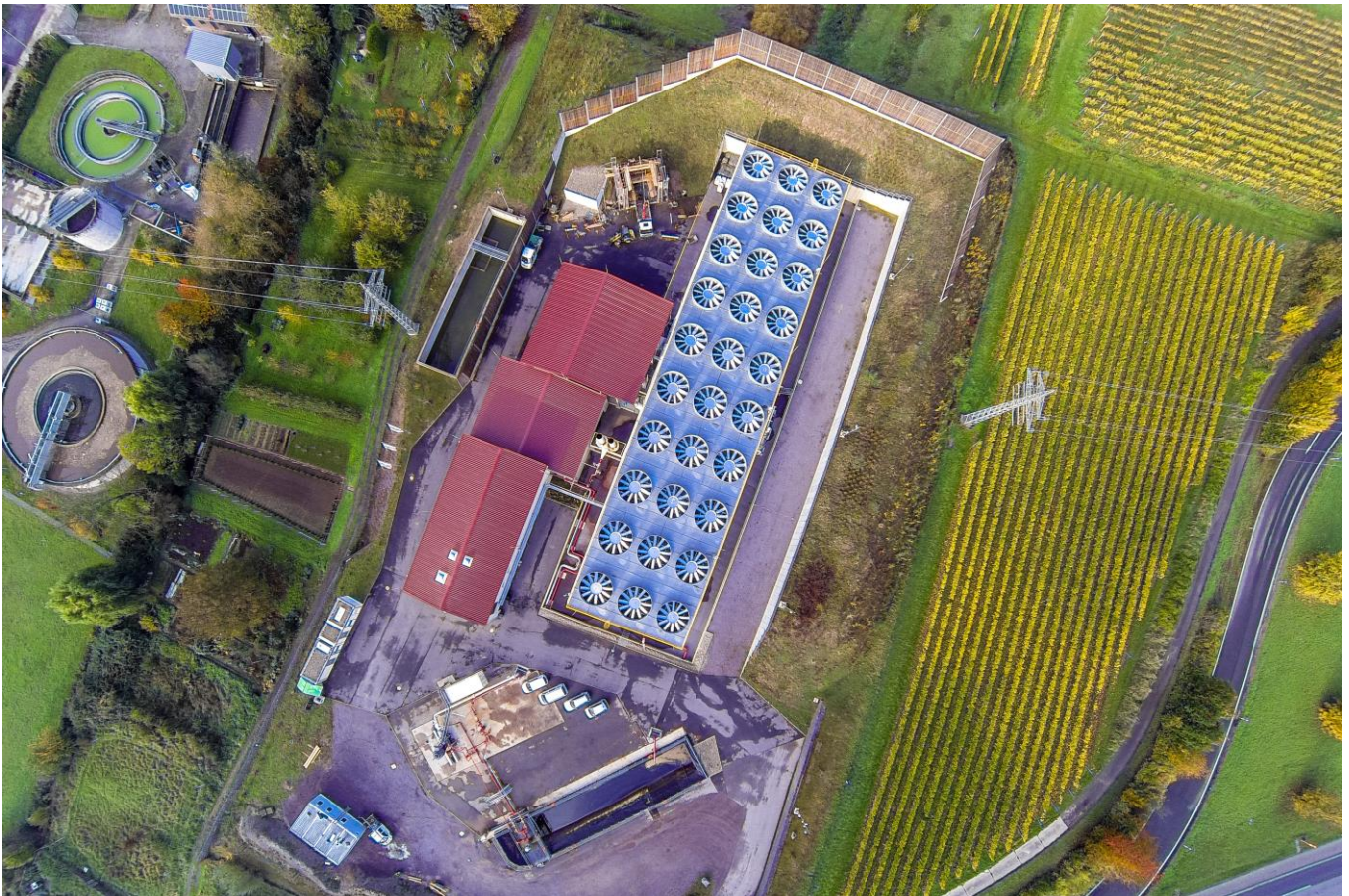
Figure 2 Vulcan's Natürlich Insheim geothermal renewable energy wells and plant
