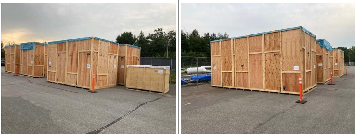
Figure 9 Pre-assembled crystallizer on its way to Vulcan's CLEOP in Höchst Industrial Park
