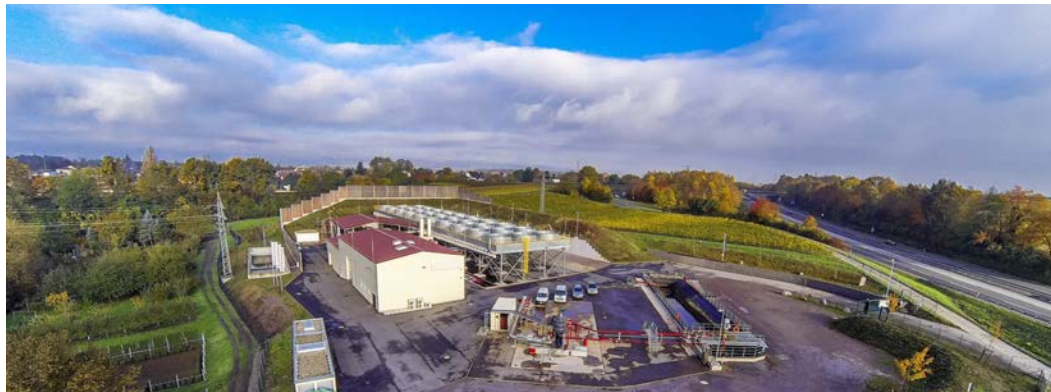
Vulcan Energy's 100% owned NaturLich Insheim, an operational geothermal renewable energy power plant in the Upper Rhine Valley, Germany.
