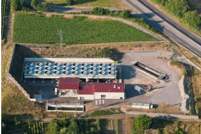
Figure 9: Aerial photograph of Vulcan's Natürlich Insheim Geothermal Plant
