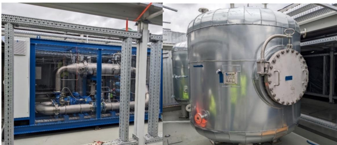
Figure 10: In-house designed lithium extraction Demo Plant, currently under construction.
