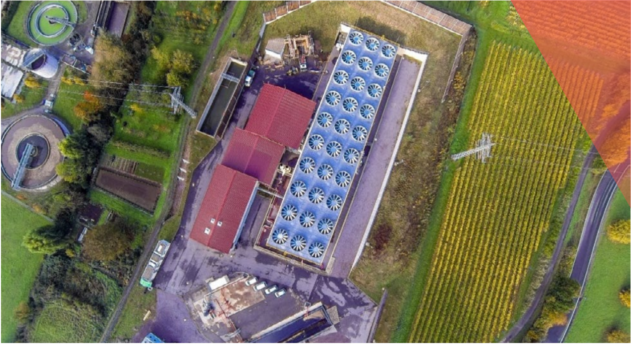
FIGURE 9 AERIAL SHOT OF VULCAN'S GEOTHERMAL POWER PLANT IN INSHEIM, GERMANY
