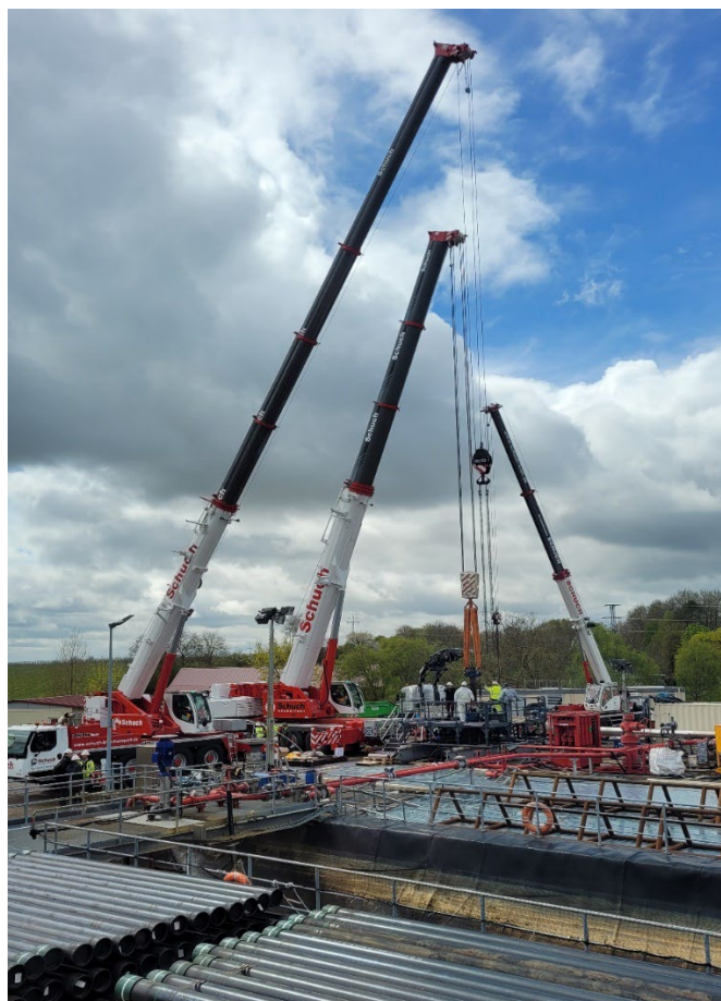
Figure 1: Natürlich Insheim - Pump replacement works.
