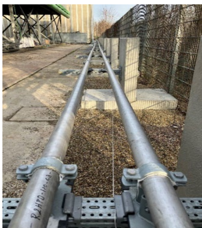
Figure 2: Brine line installation and construction progress at Vulcan's Lithium Extraction Demonstration Plant at Landau.
