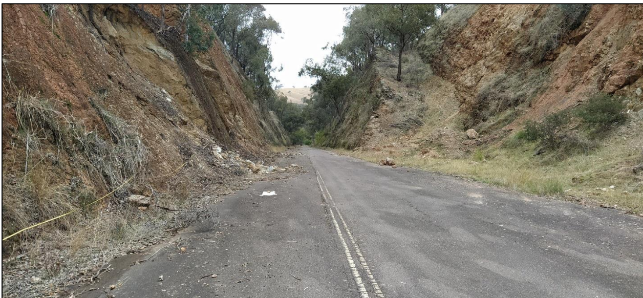
Figure 5 – The Sylvias Gap road cutting at Highway. A 100m channel sampling traverse was completed along the southern wall (left side of the image).
