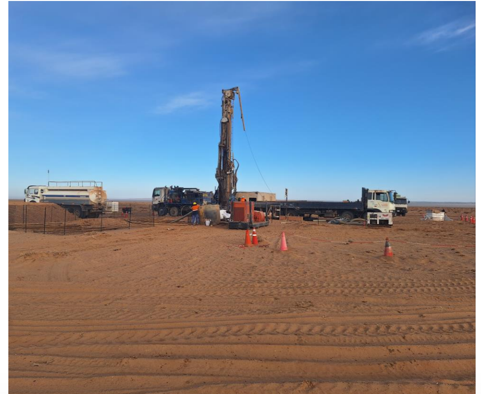
Drilling Water Monitoring Bore
