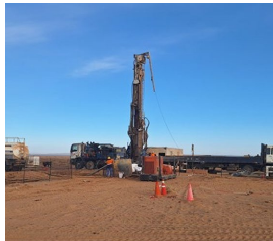
Figure 7: Water Monitoring Bore Drilling
